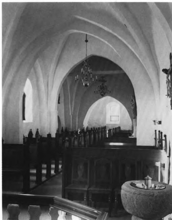
Fig. 3. Indre, set mod vest. NE fot. 1981. — Interior to the west.
